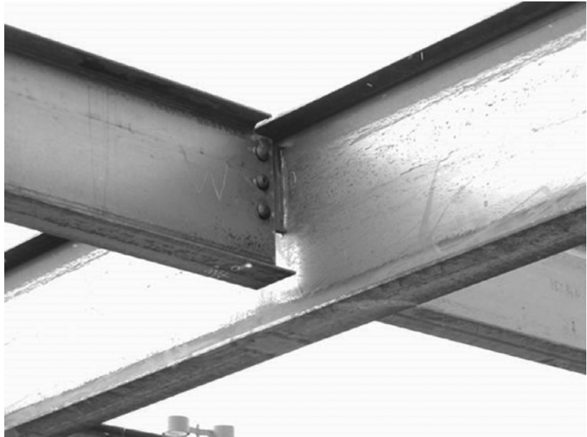
(b) Beam-to-Beam Shear Connection
