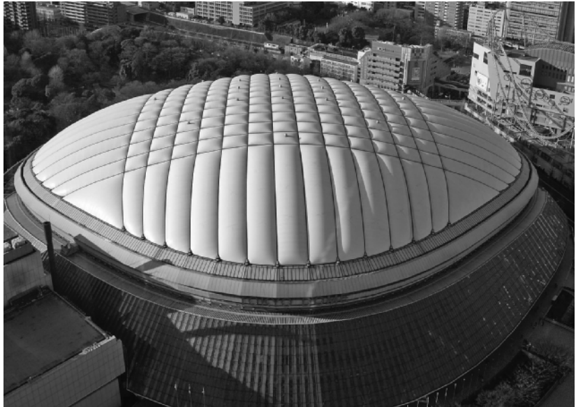
FIG. 1.6 The Fabric (membrane) Roof of the Tokyo Dome is Tensioned (inflated) by Air Pressure from Inside the Stadium © Gavin Hellier / Alamy
