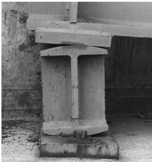
FIG. 3.5 Rocker Support Maureen M. Kassimali
