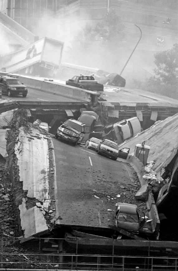
Interstate 35W Bridge Collapse in Minnesota (2007)
