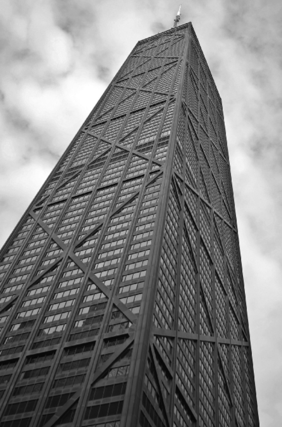
The John Hancock Building in Chicago with cross-bracing on its exterior to reduce horizontal movement due to strong winds
