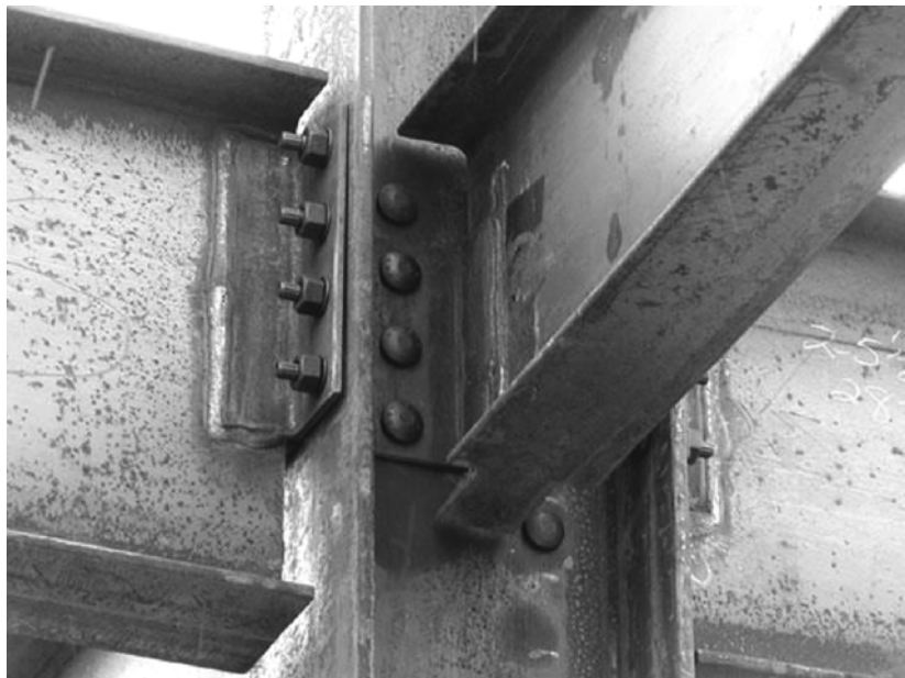
(a) Beam-to-Column Shear Connections
