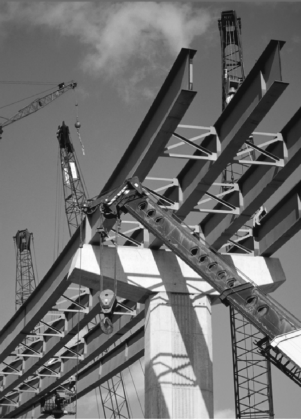
Bridge Construction on an Expressway
