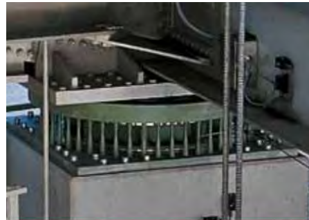
A flat surface slider with steel hysteretic dampers as installed in the Marquam Bridge, Oregon, USA.
