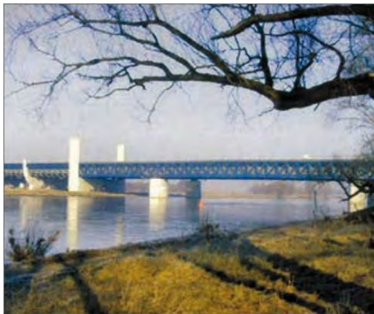
• GERMANY, MAGDEBURG -- Water Bridge shock transmission units
