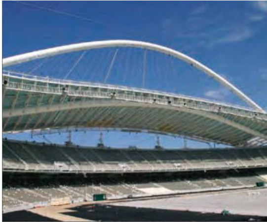
• GREECE, ATHENS -- Olympic Stadium roof special pot bearings
