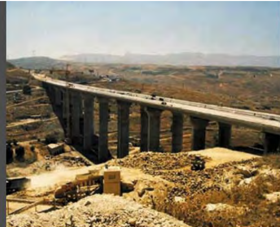
• LEBANON, BEIRUT -- Sirian Border Highway expansion joints
