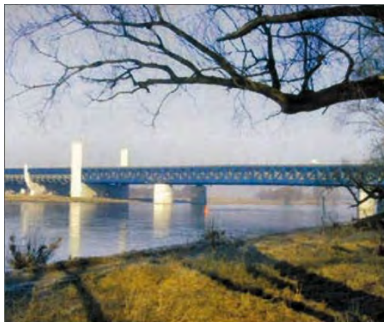
• GERMANY, MAGDEBURG -- Water Bridge shock transmission units
