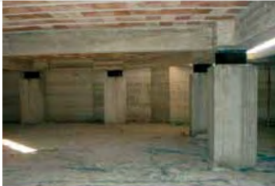
LRBs as installed in an office building in Italy.
