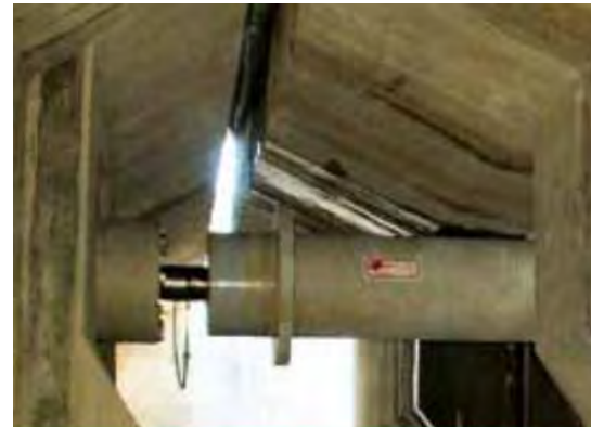
A FSD as installed in the Rio Higuamo Bridge, Dominican Republic.
