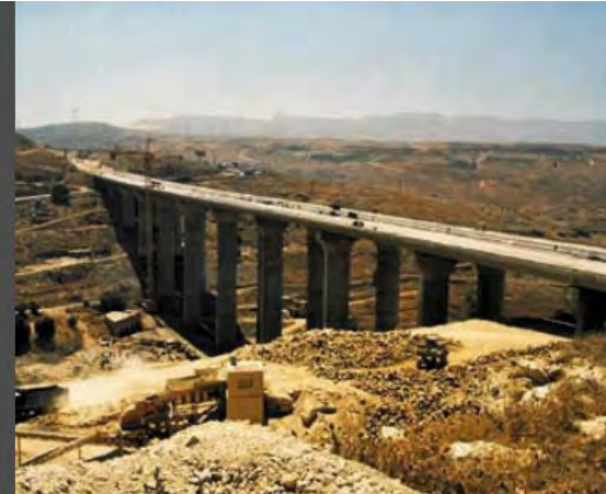
• LEBANON, BEIRUT -- Sirian Border Highway expansion joints
