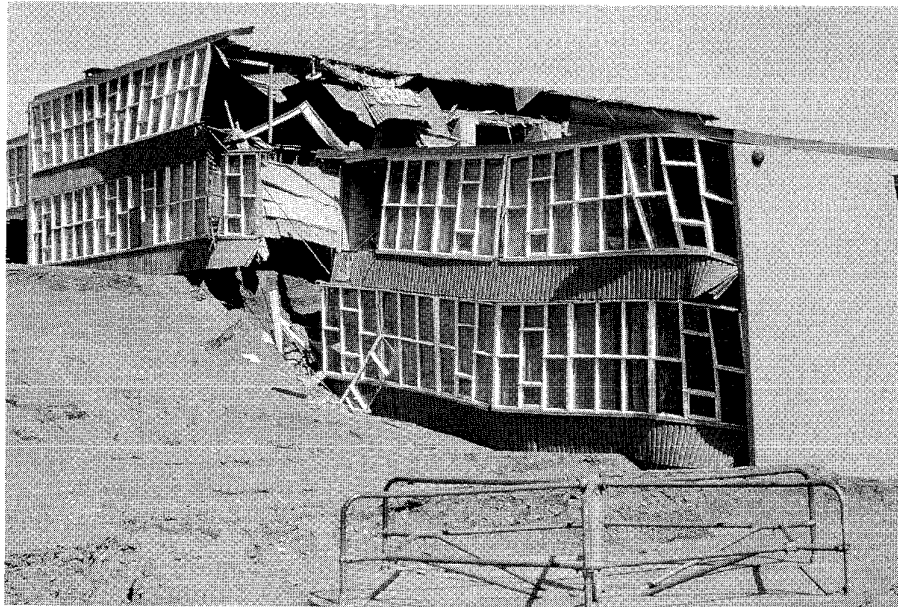
Figure 1.12 A wing of Government Hill School in Anchorage, Alaska, straddled the head scarp of the Government Hill landslide in the 1964 Good Friday earthquake (K. Steinbrugge collection; courtesy of EERC, Univ. of California).
