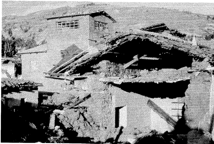
Figure 1.1 Damage to buildings in Huaras, Peru following the 1970 Peru earthquake. The adobe structures in the foreground were destroyed, but the reinforced concrete structure in the background suffered little damage (photo by G. Plafker, courtesy of USGS).
