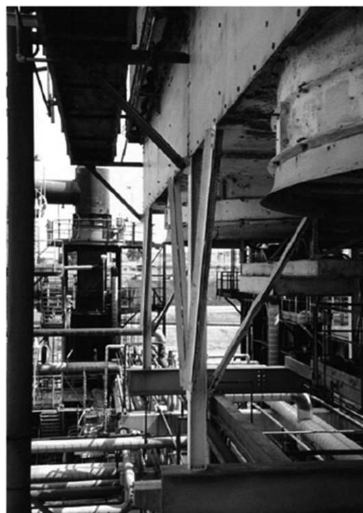
Figure C13.6-1. Fin fan elevated on integral supports.
