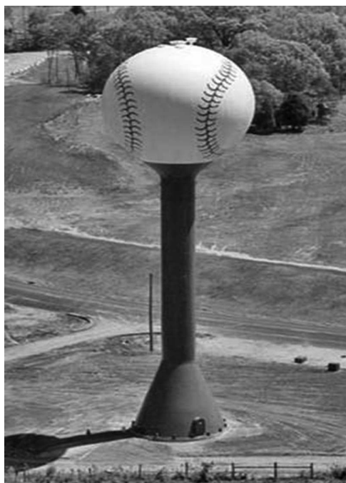
Figure C15.7-2. Small-diameter, single-pedestal steel tank.
