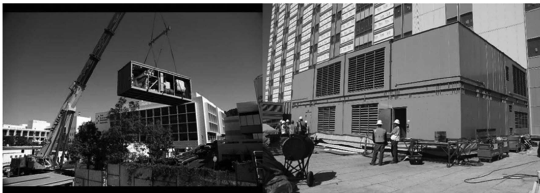
Figure C13.1-8. Premanufactured modular mechanical systems.
