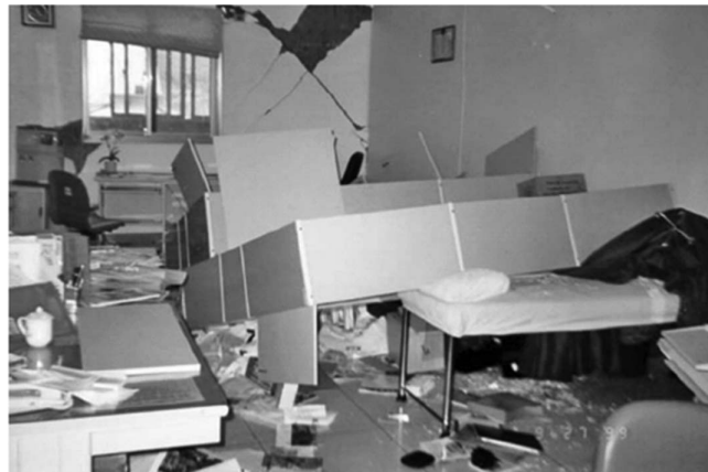
Figure C13.1-4. Toppled storage cabinets.
