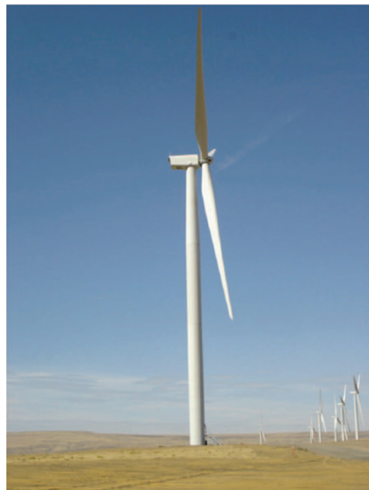
Figure C15.6-4. Typical steel tubular support structure for onshore wind turbine generator systems.
