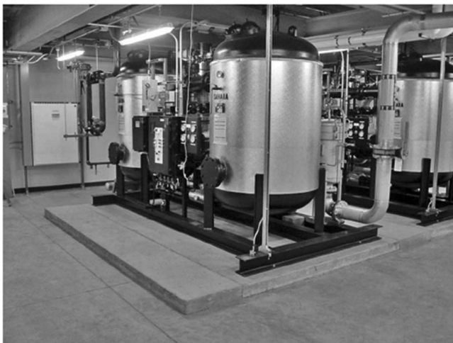
Figure C13.1-7 Skid-mounted components.
