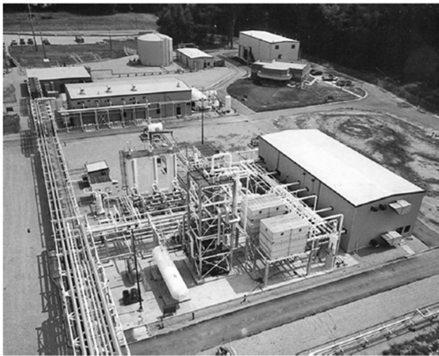
Figure C15.1-2. Steel pipe rack.
