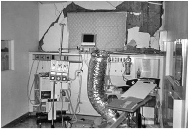
Figure C13.1-6. Collapsed duct and HVAC diffuser.
