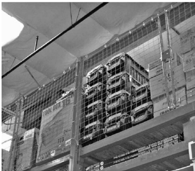
Figure C15.5-1. Merchandise restrained by netting.
