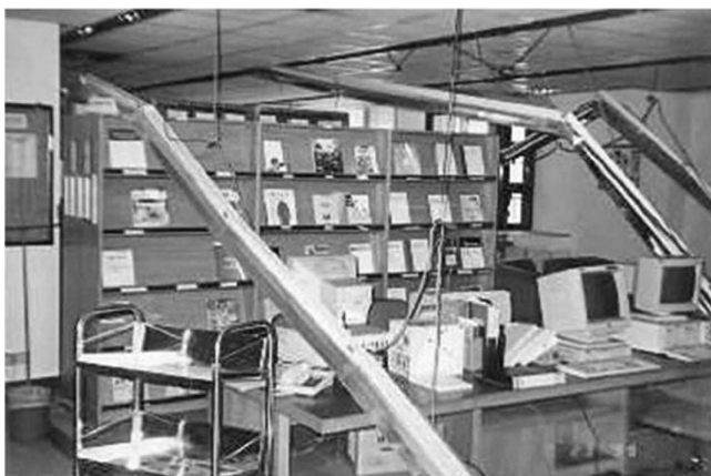
Figure C13.1-3. Collapsed light fixtures.
