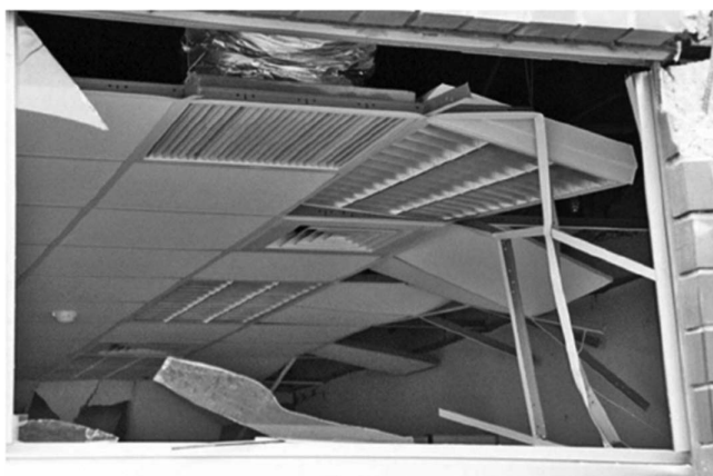
Figure C13.1-2. Damaged ceiling system.
