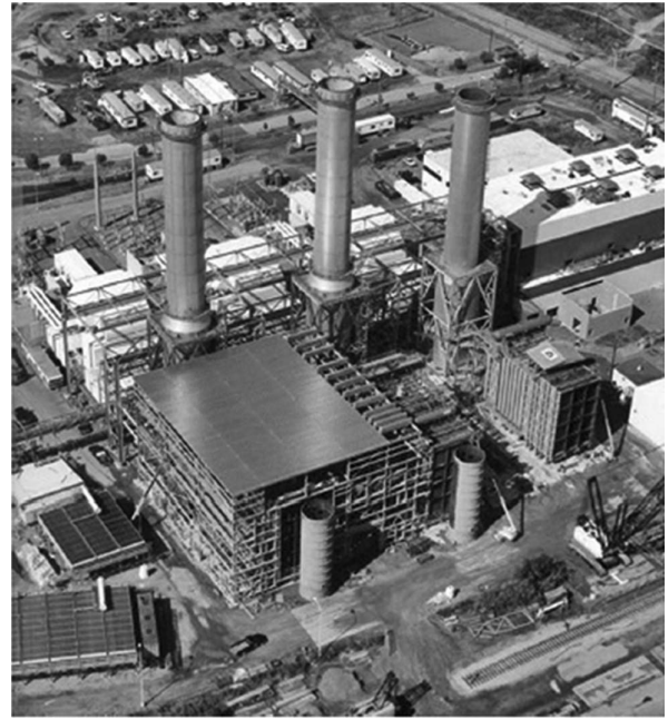
Figure C15.1-3. Heat recovery steam generators.
