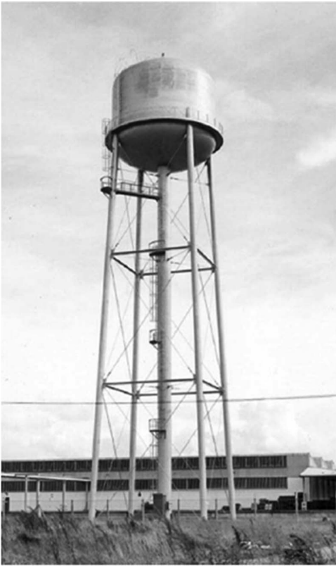
Figure C15.1-1. Steel multilegged water tower.
