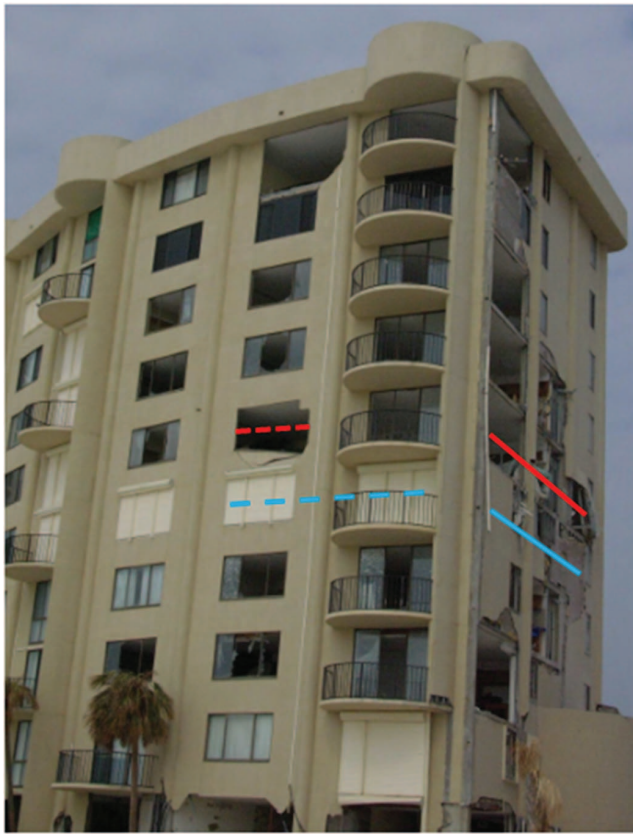
Figure C26.13-1. Glazing breaches and non-load-bearing wall failures (Hurricane Ivan). Source: FEMA (2004).
