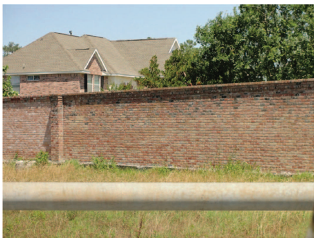
Figure C15.6-6. Typical masonry ground-supported cantilever wall.
