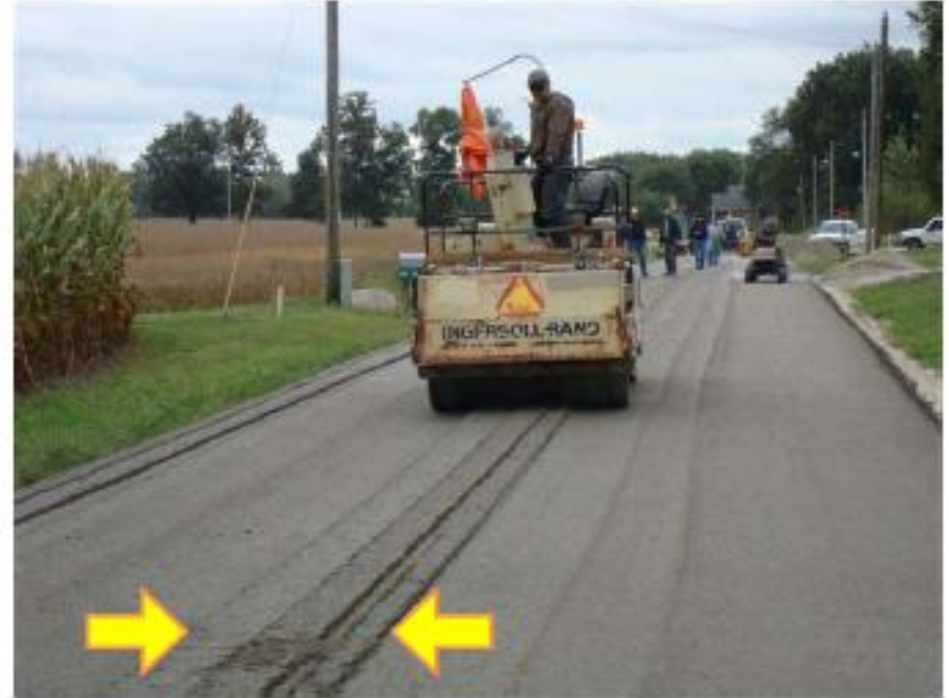
Figure 4.15 Fresh joint construction (a) Uncompact edge of the previous placement (b) the fresh joint compaction between the two adjacent lanes
