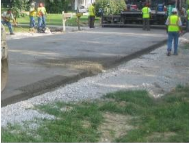
Figure 4.7 Improper moisture content:
