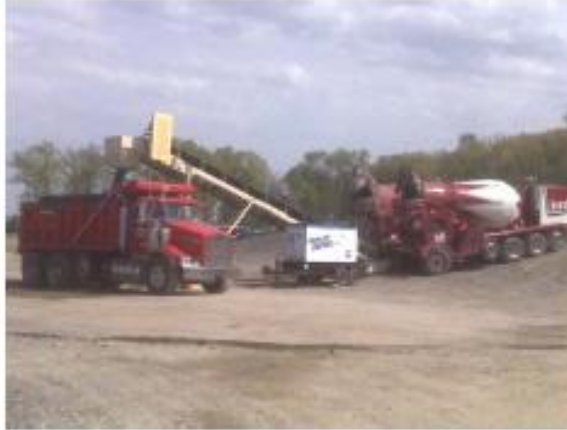
Figure 4.8 RCC is discharged from transit mixers into dump trucks
