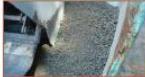
Segregation in paving hopper
