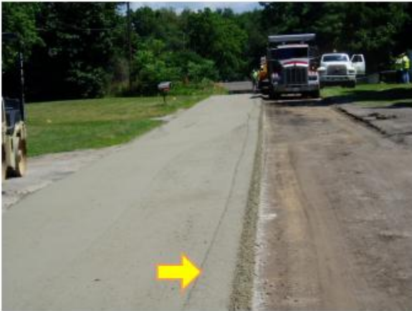
Figure 4.15 Fresh joint construction (a) Uncompact edge of the previous placement (b) the fresh joint compaction between the two adjacent lanes
