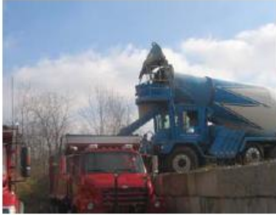
Figure 4.8 RCC is discharged from transit mixers into dump trucks
