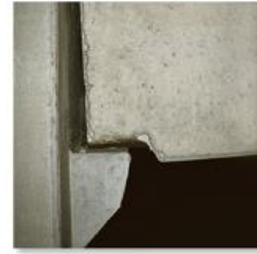
This concrete girder rests on the ledge that is assumed to act as a smooth contacting surface. (5)
