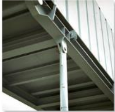
The cable exerts a force on the bracket in the direction of the cable. (1)
