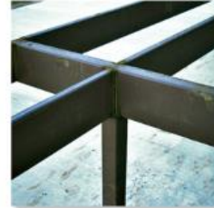
The floor beams of this building are welded together and thus form fixed connections. (10)
