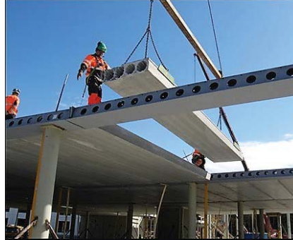
Figure 10.17(a) "Scissors" clamps used for lifting hollow-core floor units both on site and in the factory some 16 hours after casting (courtesy of Spiroll Precast Services Ltd, UK).
