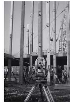
Stabilising columns with compression props and guyed ropes. The theodolite is being used to vertically align (plumb) the columns.
