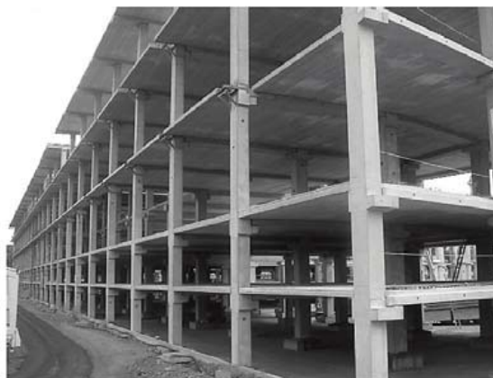
Precast concrete 'skeletal' sway frame, Europark, Rome.
