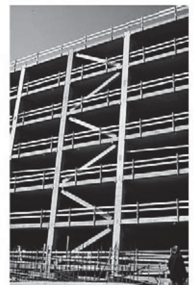
Precast concrete strut diagonal bracing.
