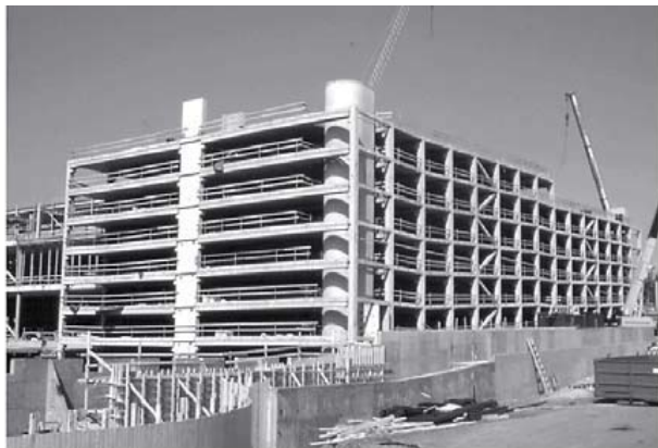
Precast concrete 'skeletal' braced frame, The 'Green Apple' retail centre and car park, Helsinki.
