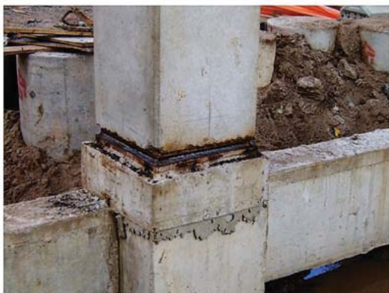
Figure 7.138 Steel base plate fully welded to cast-in plate in pile cap (courtesy of T&A Prefabricados, Recife, Brazil).
