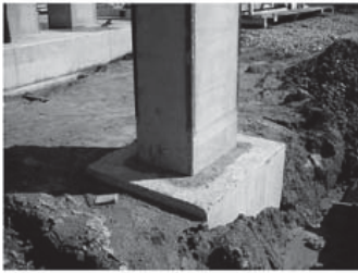
Column-to-foundation connection using a grouted pocket.
