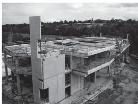
Forming the stability of multistorey frames using discrete structural elements. (Courtesy of Westkon, Melbourne, Australia.)
