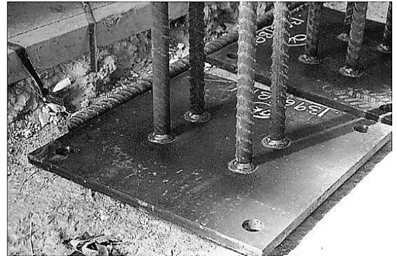
Figure 10.54 Column steel base plate with starter bars.
