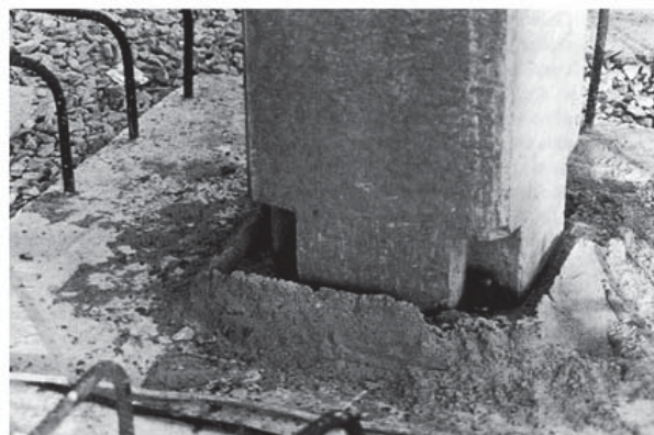
Figure 7.137 Column-to-foundation connection with flush base plate.
