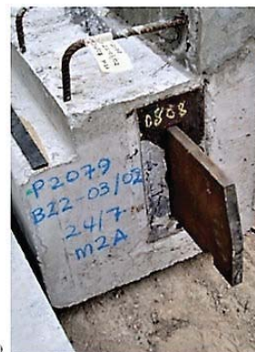
Figure 7.69 (a) Sliding plate connector steel plate is expressed from the beam after casting, and (b) is received into the steel box slots in the column.
