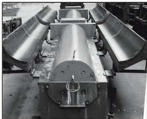
Manufacture of high-strength circular columns. (Courtesy of Ergon, Lier, Belgium.)
