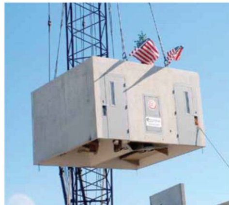
Fig. 1.2.16 A precast concrete double-cell module is lifted into place, complete with furnishings installed.
