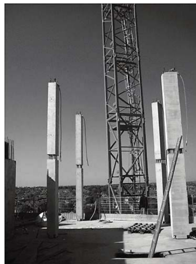
Precast columns with openings for in situ stitching to beam and/or slab connections. (Courtesy of HSP Consulting, Nottingham, UK.)
