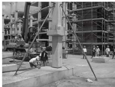
Stabilising columns with compression props.
