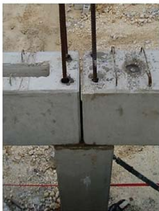
Figure 7.43 (a) Discontinuous pinned jointed beam-to-column connection; (b) close-up view.
