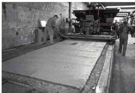
Figure 5.55 Manufacture of double-tees. (a) Using concrete pouring arms and (b) using concreting train.
