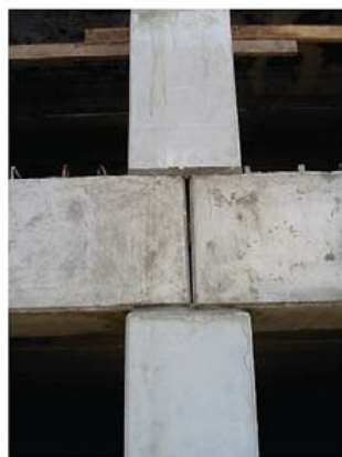
Figure 7.43 (a) Discontinuous pinned jointed beam-to-column connection; (b) close-up view.
