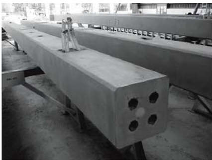
Manufacture of precast-reinforced concrete column. (The sleeves receive waiting rebars on site.)
