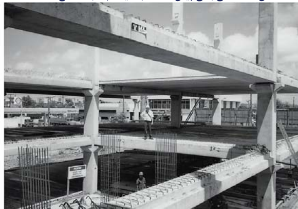
Precast concrete 'skeletal' known as 'semi-rigid' frame, Recife University, Brazil.
