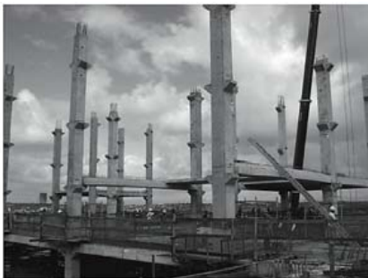
Five-storey-tall precast columns with corbels. (Courtesy of T&A, Recife, Brazil.)
