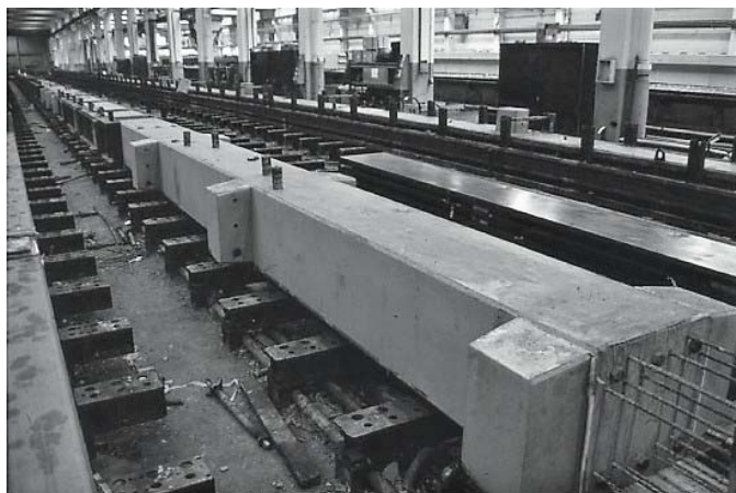
Manufacture of (lightly) prestressed concrete column.
