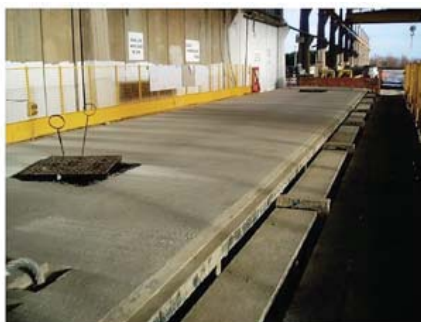
Figure 5.57 Surface finishes to the tops of double-tee slabs are tamped rough.
