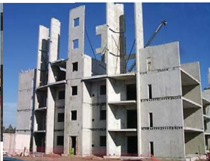
Forming the stability of multistorey frames using discrete structural elements. (Courtesy of Westkon, Melbourne, Australia.)
