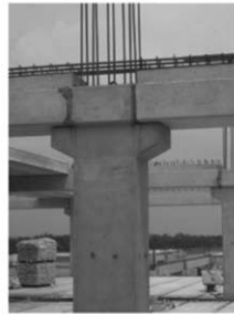
Figure 9.5 Precast concrete column corbel.
