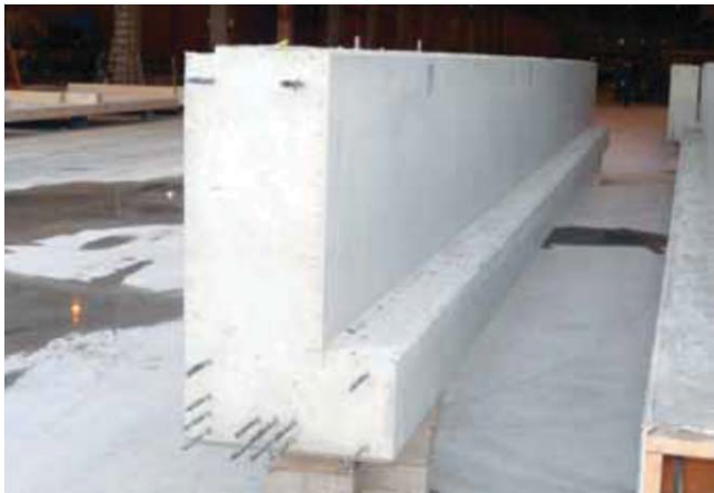
ledger beam(L shaped beam)
