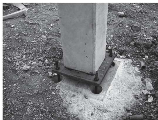
Figure 10.4 Column-to-foundation connection using extended steel base plate.
