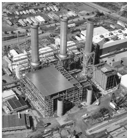
FIGURE C15.1-3 Heat recovery steam generators
