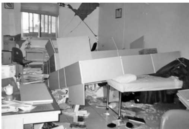
FIGURE C13.1-4 Toppled Storage Cabinets
