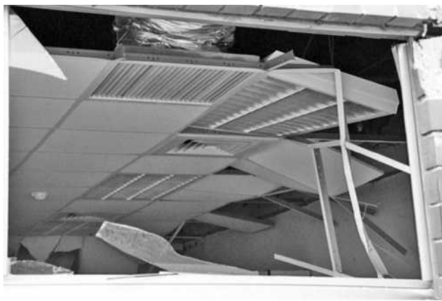
FIGURE C13.1-2 Damaged Ceiling System
