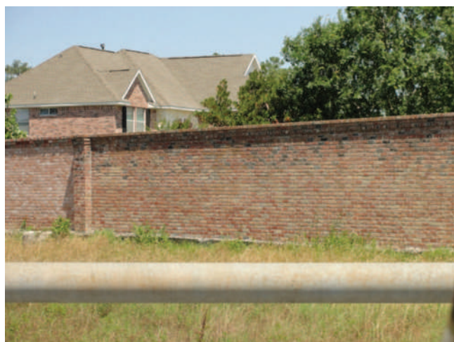
FIGURE C15.6-4 Typical Masonry Ground-Supported Cantilever Wall
