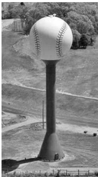
FIGURE C15.7-2 Small-diameter, single-pedestal steel tank
