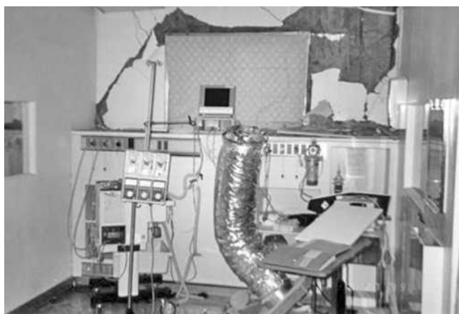
FIGURE C13.1-5 Collapsed Duct and HVAC Diffuser
