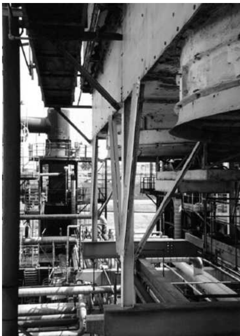
FIGURE C13.6-1 Fin Fan Elevated on Integral Supports
