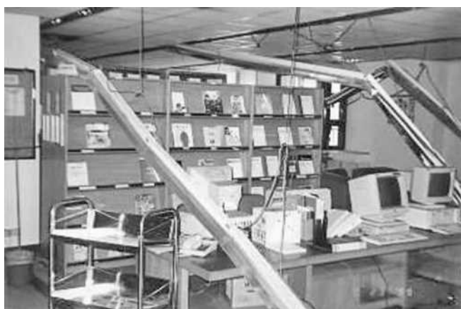
FIGURE C13.1-3 Collapsed Light Fixtures
