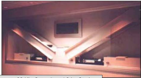
62 Dampers: 30 Kip Capacity, +/-2 in. Stroke
