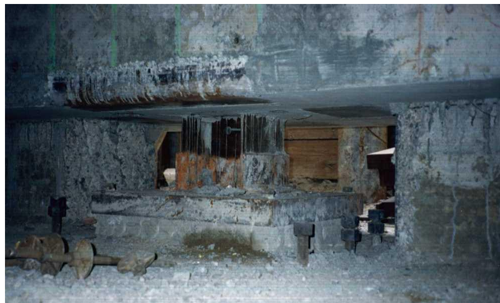
Cutting hole for jacks and column removal
