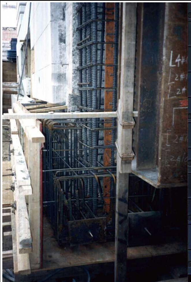
Cutting hole for jacks and column removal
